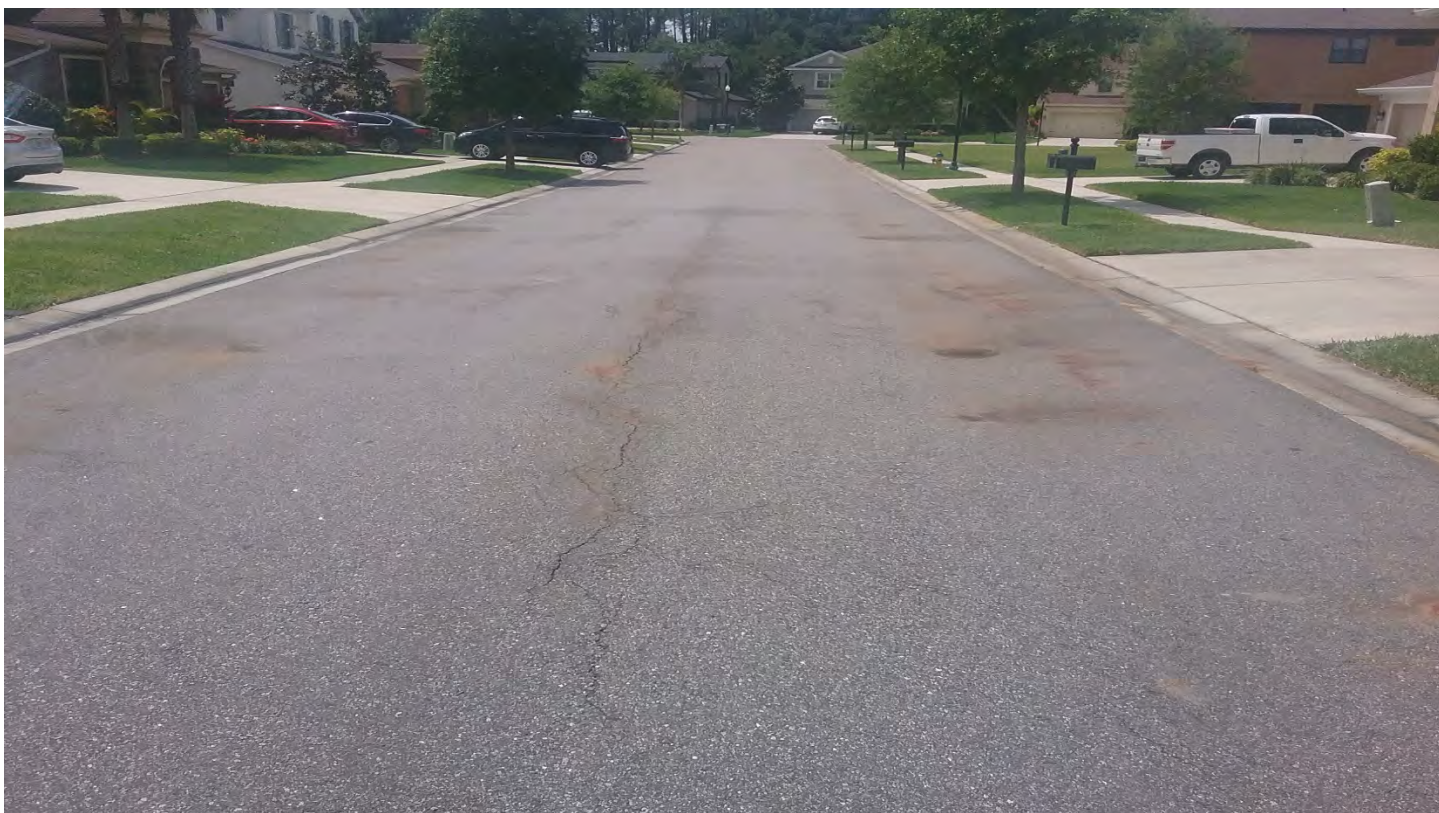
There was only minor water seepage through the asphalt on Cottage Glen Lane.
